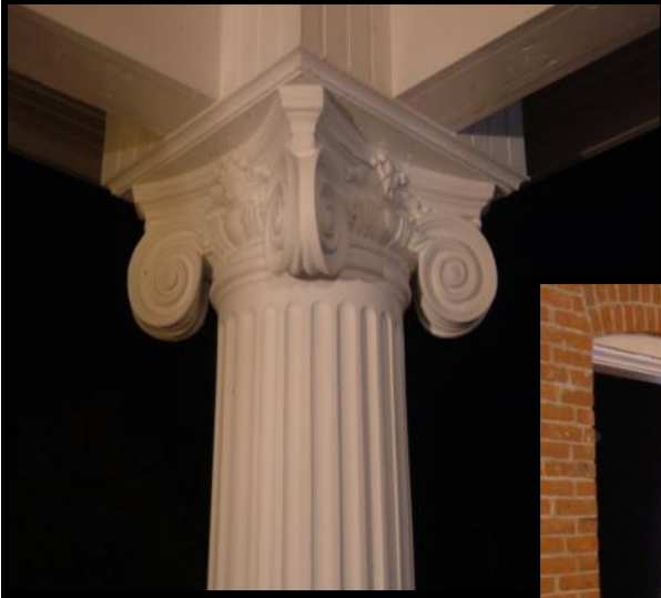
Exterior porch column
